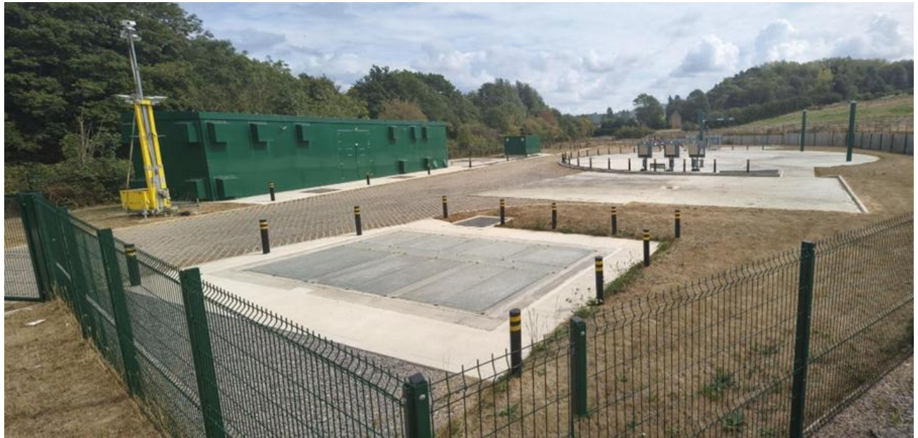
Ebley Meadows stormwater storage installation, Stroud.
