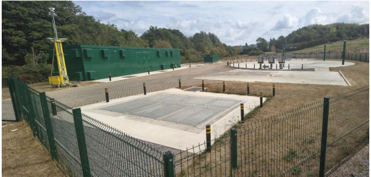
Ebley Meadows stormwater storage installation, Stroud.
